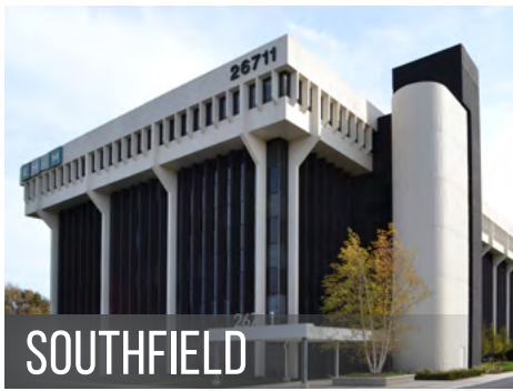
SOUTHFIELD 26711 Northwestern Highway
